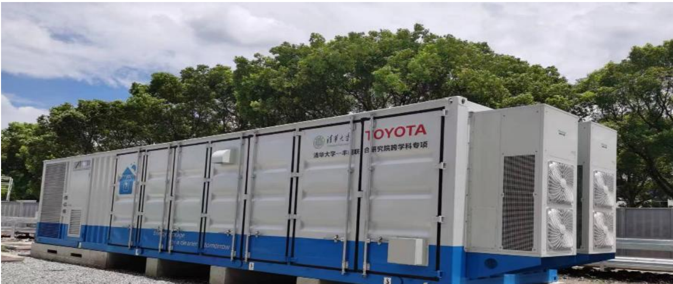
Shanghai Capacity--1000kW/2788.5kWh
